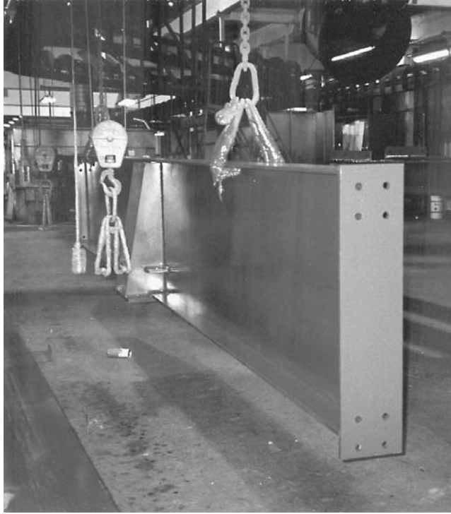
FIGURE 9.1 Shop primer is applied to a segment of primary frame.
